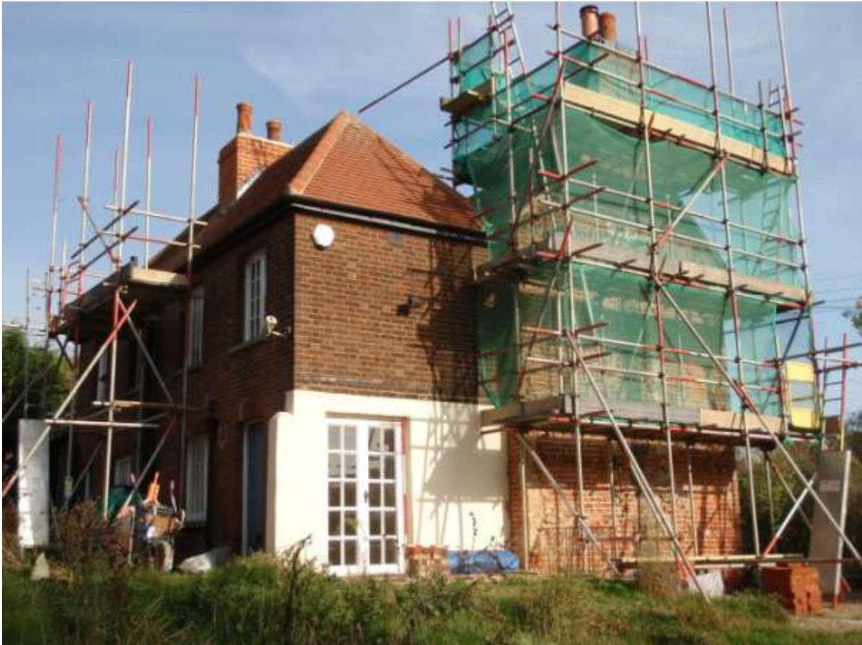
Plate 5. West (rear) and south elevation showing new roof (looking north-east)
