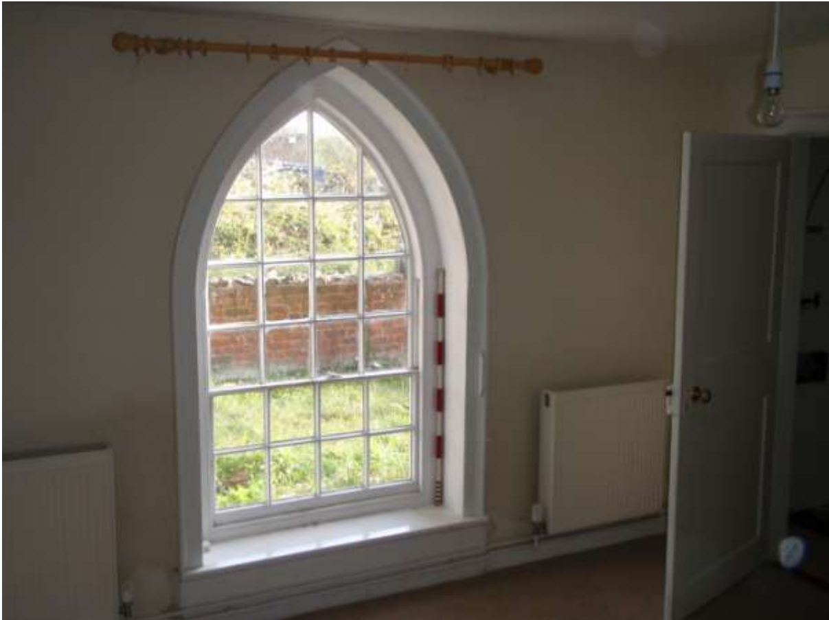
Plate 11. Living Room (2) interior (looking south-east)
