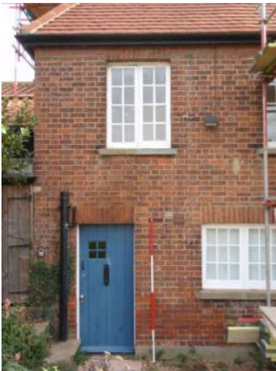
Plate 6. Detail of west (rear) elevation (looking east)
