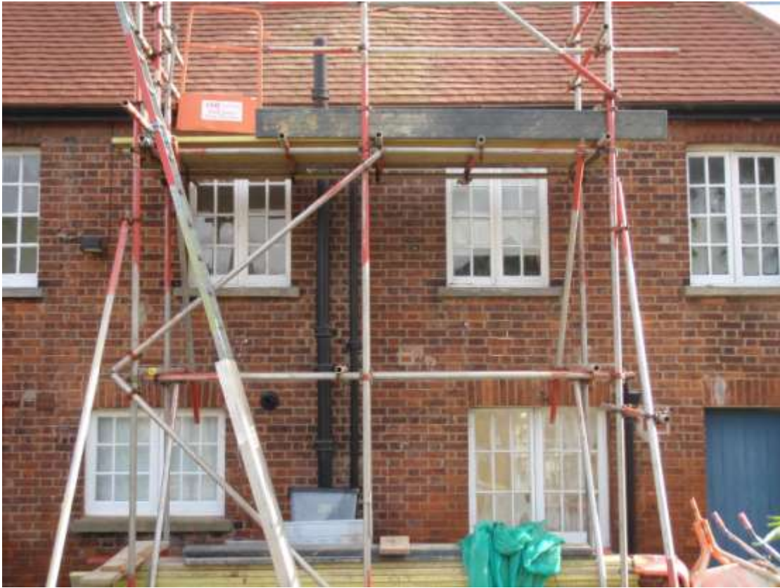
Plate 7. Detail of west (rear) elevation phase 2 (looking east)
