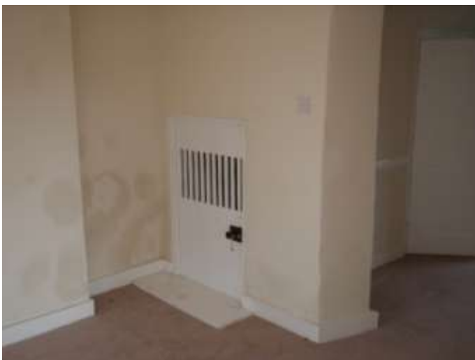
Plate 14. Detail of Utility Room (5) showing doorway to cellar
