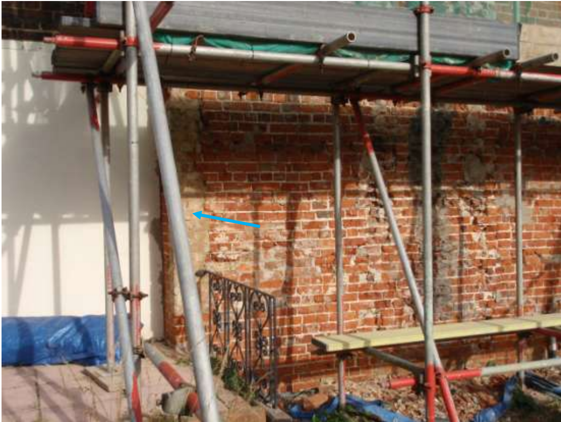
Plate 8. Detail of south elevation phase 1 showing damaged brickwork of demolished 'bake-house')
