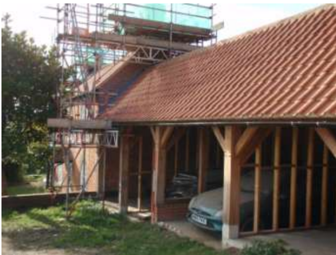
Plate 2. Front elevation of the new four bay barn (looking west)
